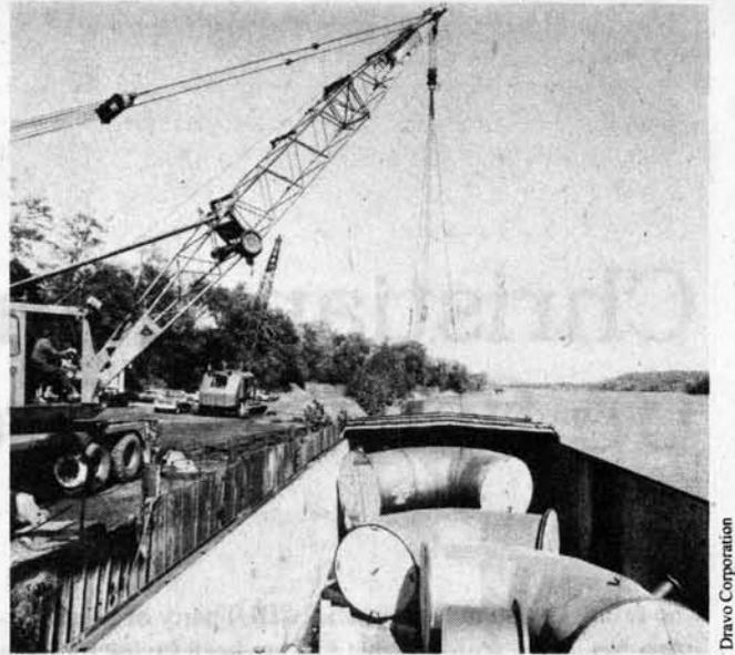
*Pipes for water intake at a nuclear power project in the Philippines. The Kra Canal will boost Thailand's nuclear industry.*
