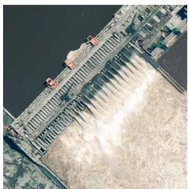
voirs. I can tell you very briefly, because if I have to go into the details it may take a couple hours. This reservoir will be silted up; but the percentage of sediment in the reservoir would only take away, roughly, 40% of the reservoir capacity, in the very long term; 60% of the capacity of the reservoir will be preserved in perpetuity.
