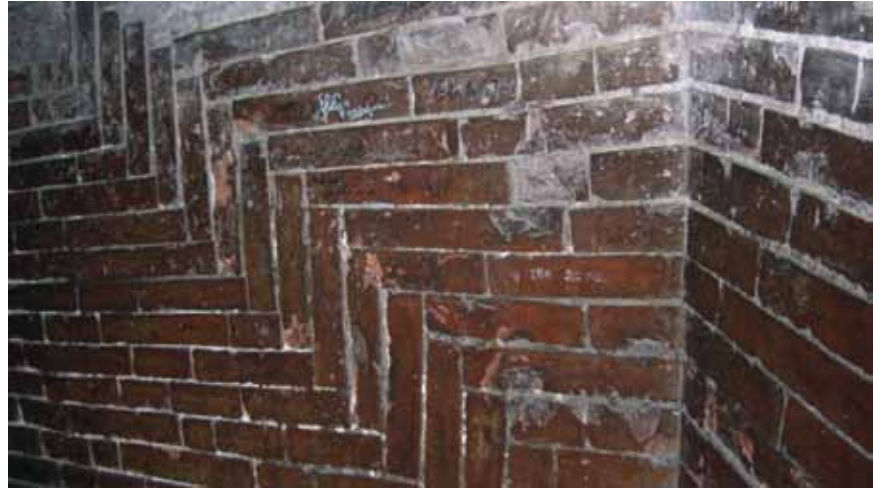
The herringbone brickwork in the space between the inner and outer domes.
