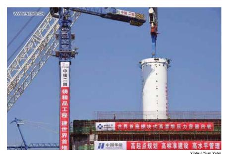
To deal with trans-Atlantic corruption and degeneration, a great change will be necessary which will be located in places like Russia and China. Here, the pressure vessel of a high-temperature gas-cooled reactor is being installed March 20 at the Huaneng Shidao Bay nuclear power plant in China's first fourth-generation nuclear energy system.
