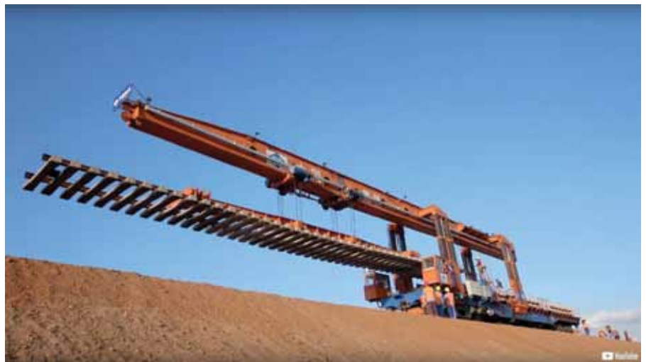
Track-laying machine at work on Mombasa-Nairobi railway.
