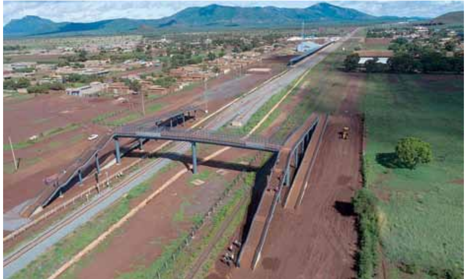
Pedestrian bridge near the Emali station of the Mombasa-Nairobi railway. It has been designed so that it can also be used as a livestock overpass.
