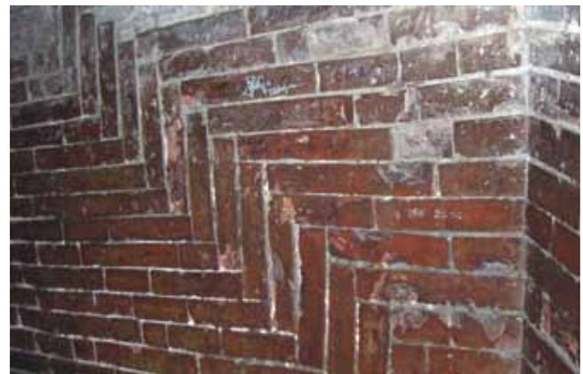
*Brunelleschi's use of a herring-bone pattern of the brickwork, in the space between the inner and outer domes, allowed them to self-reinforce as they were being laid.*
