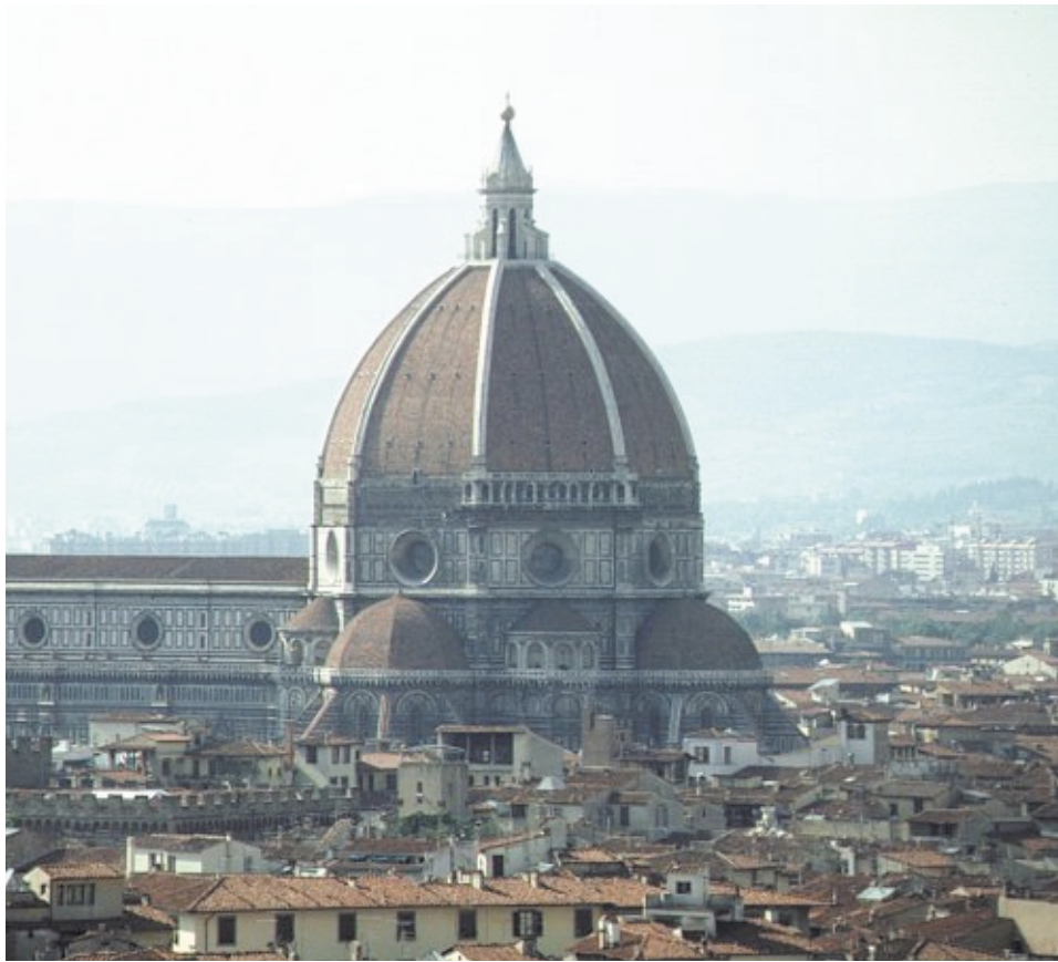
The Cupola on Florence Cathedral. Brunelleschi used “hanging chains” (catenaries) as guides during construction. Inset: Filippo Brunelleschi.
