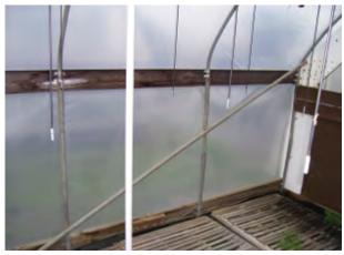
Diagonal bracing should be included in all greenhouses to prevent racking of the frame.
