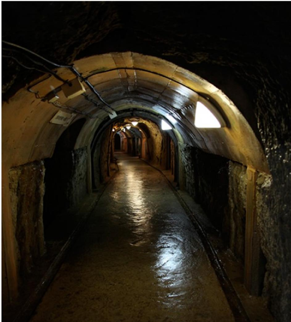
Photograph of the bunker corridor. This is concrete lined, which is interesting in that's very different to the log-based tunnels on Ie Shima made by the same army in the same time period. No concrete for Ie Shima. Just lumber.
